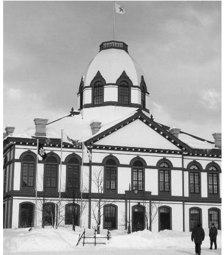
Restored main office building of Kaitakushi (2005) Source: Kinori (Wikimedia Commons)
