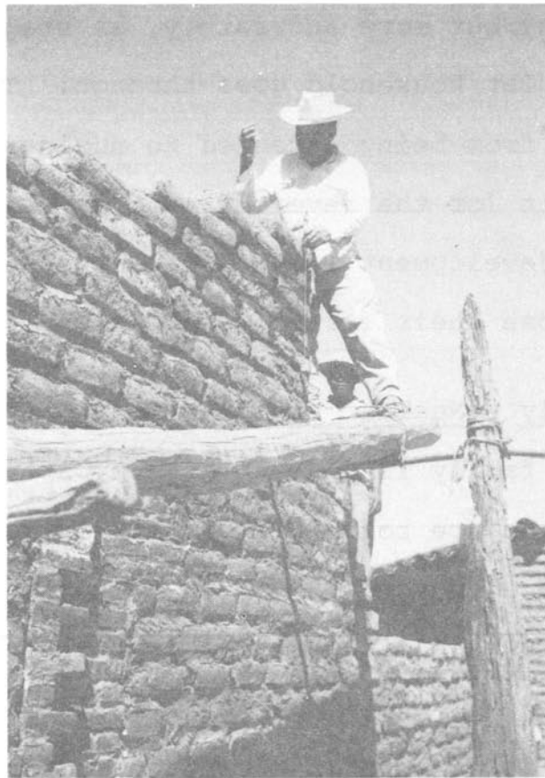
Adobe wall being constructed. Matatlan, Oaxaca, 1967.
