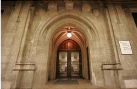
Figure 3: Original main entrance to the library
