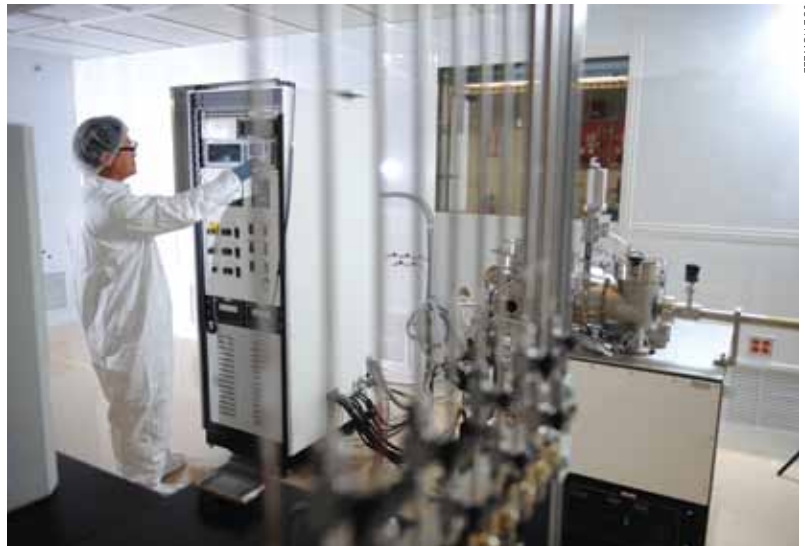
VINSE recently renovated the air-handling and toxic gas monitoring equipment in its clean room, thanks to an American Recovery and Reinvestment Act (ARRA) grant. Research Assistant Professor of Electrical Engineering Bo Choi works at the eBeam evaporator in the room.
