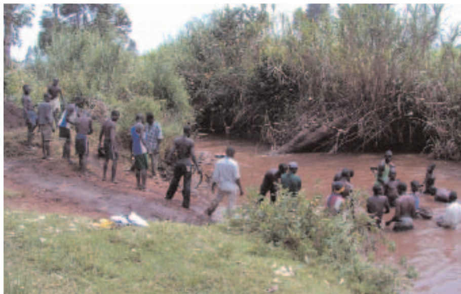
A team of villagers dredges sand from a nearby river to make the clinic foundation.
