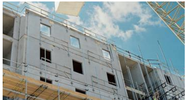
(b) During construction
