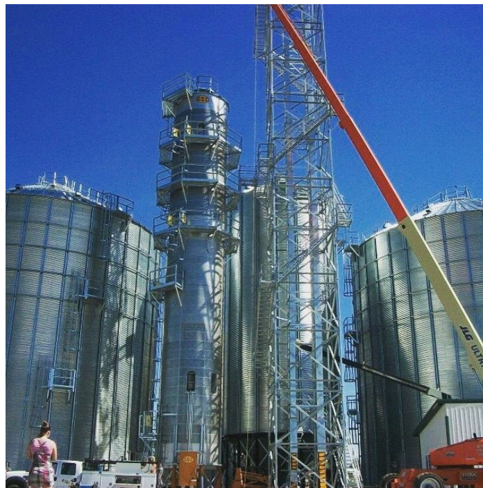
Figure 3: Grain Storage Bins
