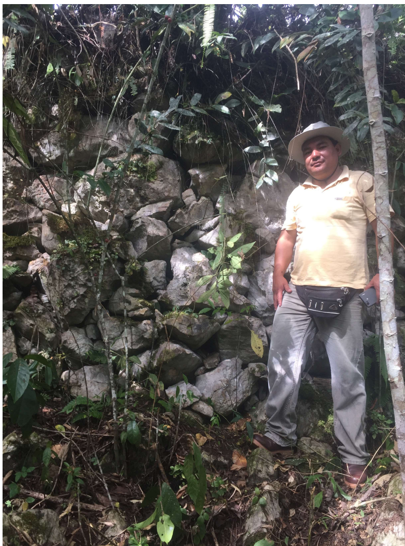
Figure 4.5: Retaining wall documented during 2013 survey, Lic. Willy Chiguala Villanueva for scale.
