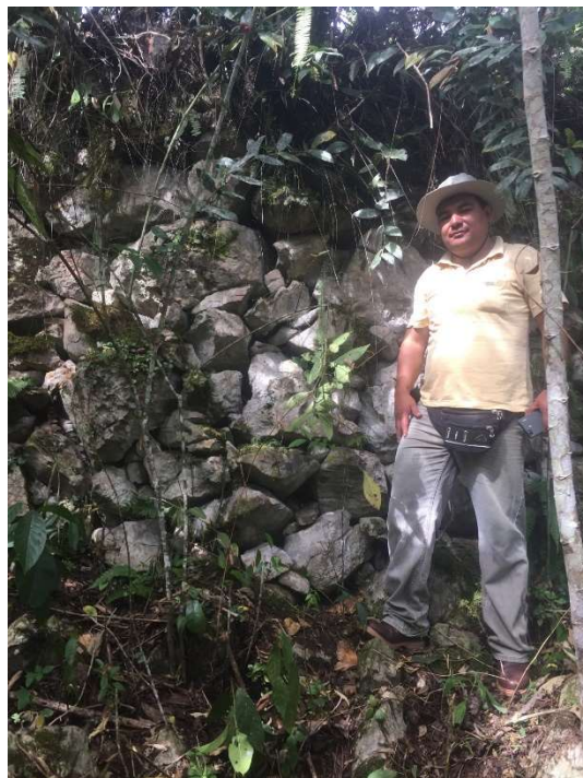
Figure 5.22: Terrace wall south of Platform 3
