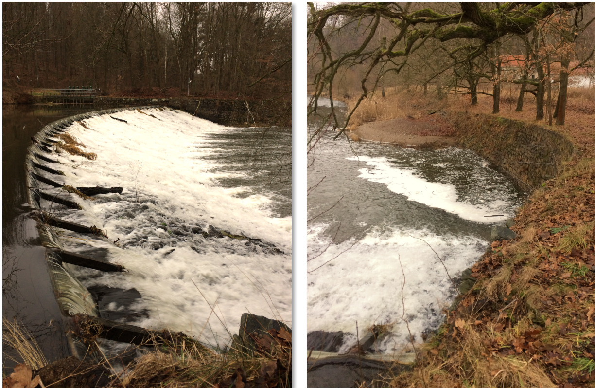
Figure 4. (Left) The arch of the Gersdorf weir, photographed by the author in December 2018. The sluice that opens to a canal, which powered three water wheels, is faintly visible on the opposite bank. (Right) Facing downstream, the curling “bulwarks”— Vestungswerke , Schützwerke , or Eißküsten , as Mende variously called them—of the Gersdorf weir, which have indeed survived to the present.
