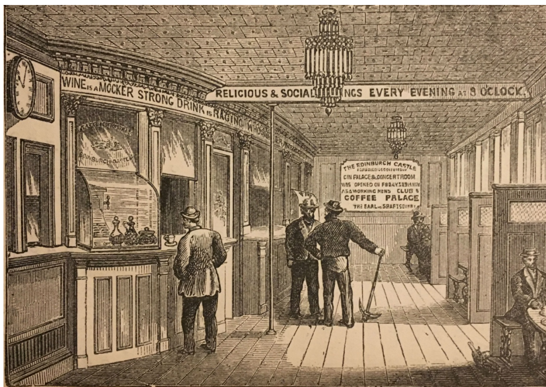
Figure 5.3. Interior of the Edinburgh Castle Coffee Palace.
