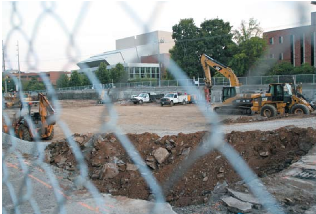
Construction for the new parking garage at Highland Quad, September 8, 2008.
