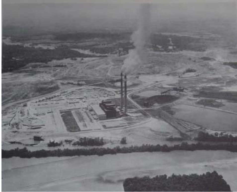
Figure 6.4b: Paradise Steam Plant (aerial) – An aerial photograph of Paradise Steam Plant circa 1964. Source: TVA, The Paradise Steam Plant: A Report on the Planning, Design, Construction, Costs, and First Power Operations of the Initial Two-Unit Plant, Technical Report No. 37 (Knoxville, TN: TVA, 1964), 26, copy in NARA-SE, RG 142, OEDC, Box 636.
