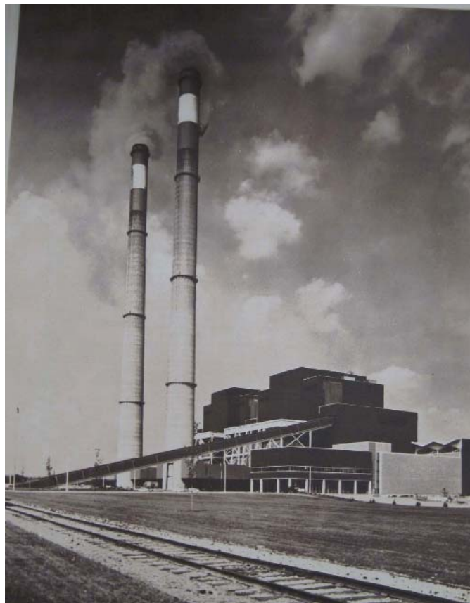
Figure 6.4a: Paradise Steam Plant – A ground level view of Paradise Steam Plant circa 1964. Source: TVA, The Paradise Steam Plant: A Report on the Planning, Design, Construction, Costs, and First Power Operations of the Initial Two-Unit Plant, Technical Report No. 37 (Knoxville, TN: TVA, 1964), frontispiece, copy in NARA-SE, RG 142, OEDC, Box 636.
