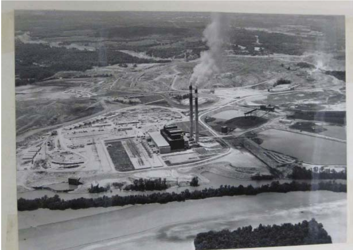
Figure 2.6: Paradise Steam Plant circa 1964. Source: TVA Division of Engineering Design, "Paradise Steam Plant: Final Design Report," Report No. 40-200, May, 1964, interior leaf, NARA-SE, RG 142, OEDC, Box 631.
