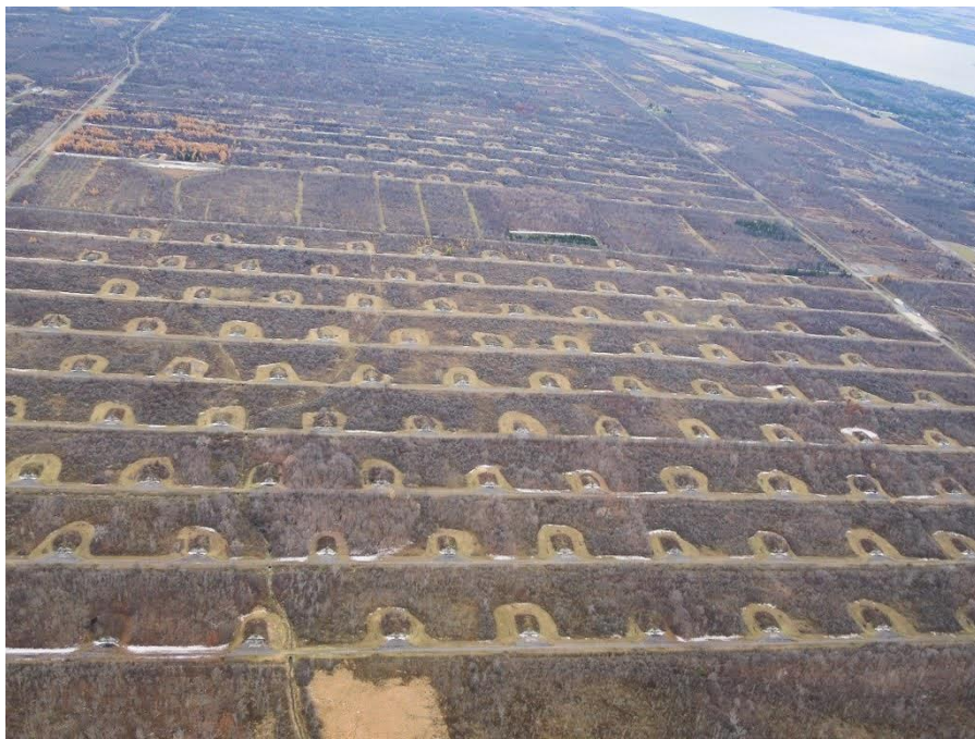
Figure 4: Seneca Army Depot, Aerial Photograph of Munitions Bunkers, http://warrior481.blogspot.com/2014/11/seneca-lake-exploration.html
