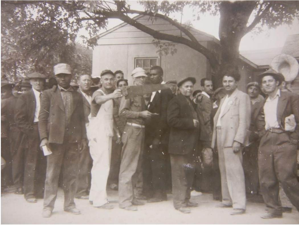
Figure 22: Workers at the Seneca Army Depot construction site, P.B. Oakley Collection, Geneva Historical Society.
