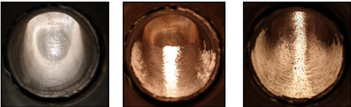
Figure 3-14: Pipe elbow before (left) during (middle) and after (right) material removal
