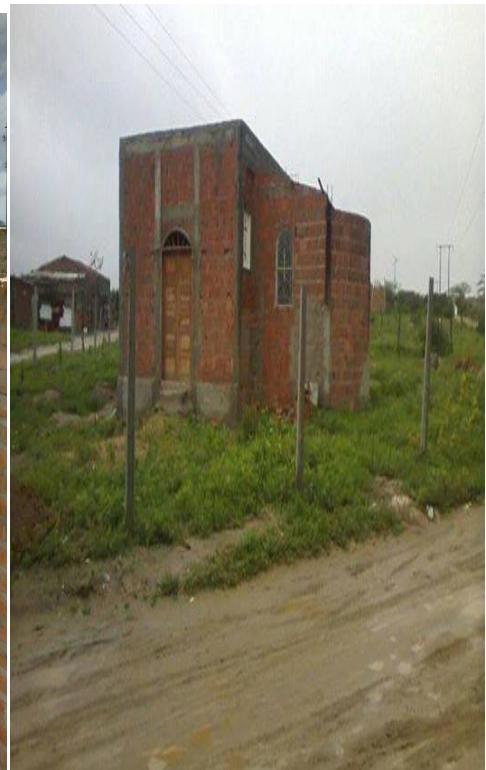
Figure 18: The construction of Saint John Chrysostom Parish in June 2017.
