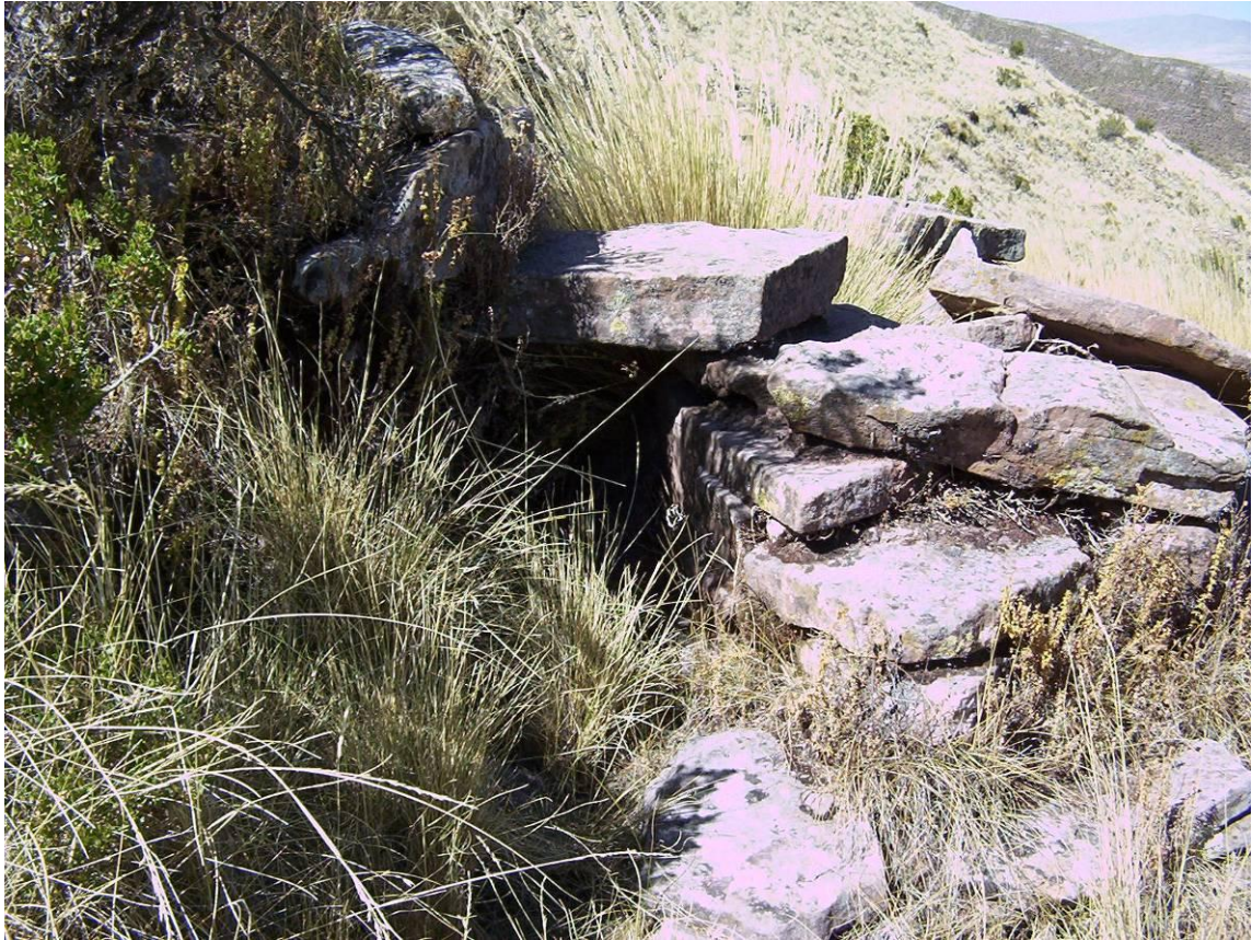
Figure 23: Structure E114, showing low lintel
