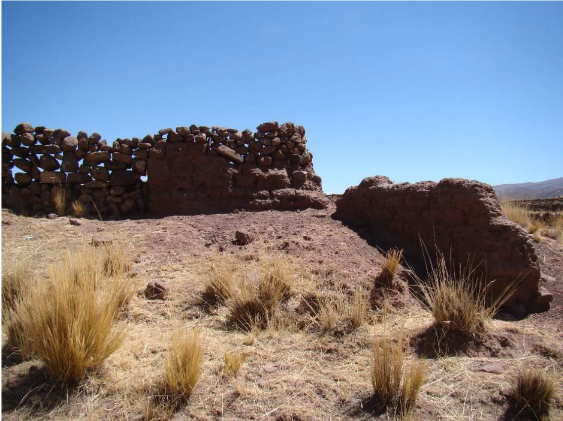
Figure 58: Entrance to the colonial church at Ch'auca de Khula Marka. Original church walls are built from adobe. Stones (current construction) fill the doorway.
