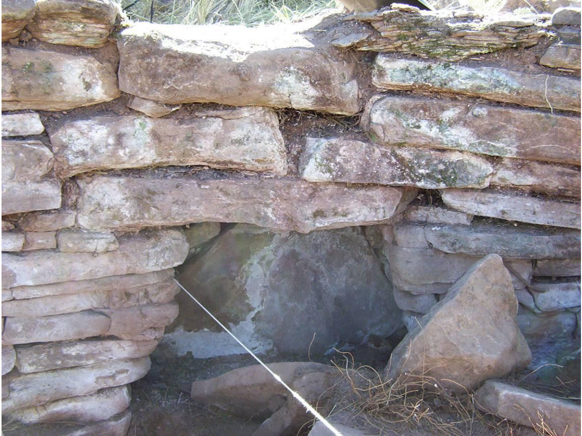
Figure 25: A typical niche in the north wall of structure E120 (U3.1)
