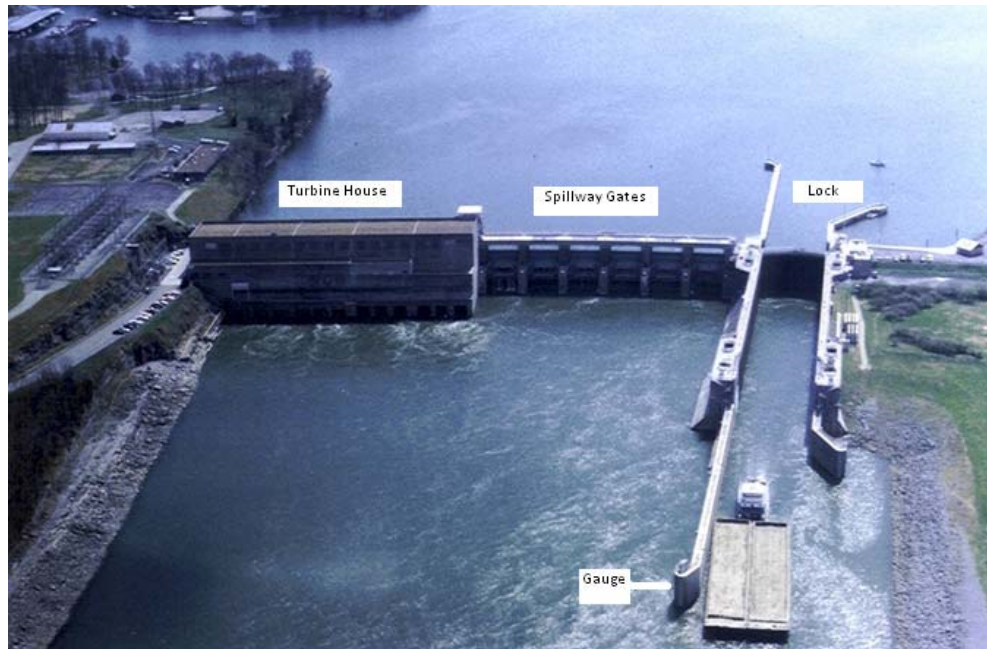
Figure 6-22. Old Hickory Lock and Dam.
