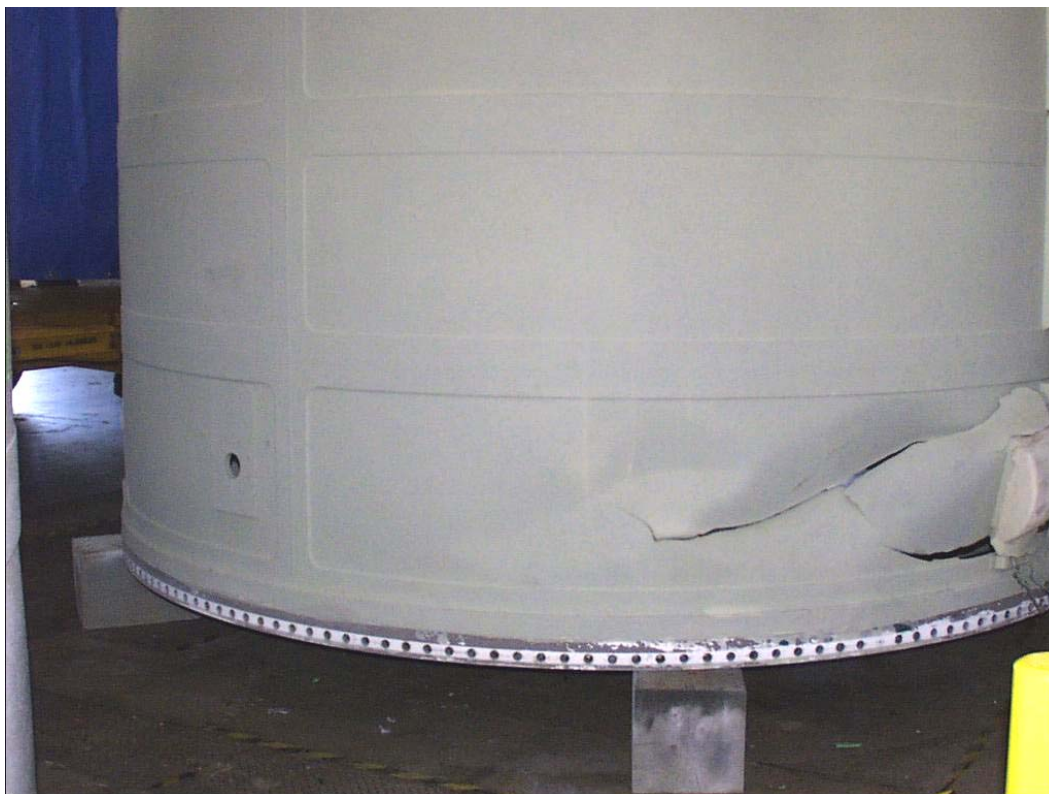
Fig. 5.18 – Buckled patterns on SRB forward skirt
