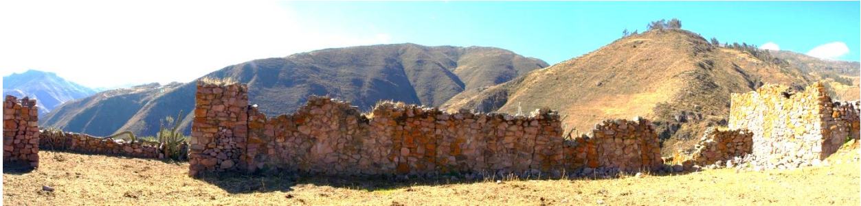
Figure 7.36: Panoramic view of the stone pillars in the Semi-Circular plaza of Canchaje (photograph by PASL 2011).
