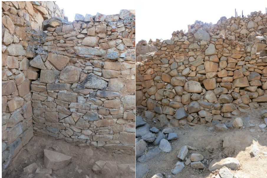
Figure 6.44: Details of masonry in the Rectangular Residential Compound. Notice the height of the walls, and that there is a better fit between the small angular stones and a tendency towards horizontality in the way in which the stones were laid. There are some medium stones in the middle, yet they are smaller in size than those of the Circular Residential Structures. The mortar is better preserved (photographs by PASL 2015).
