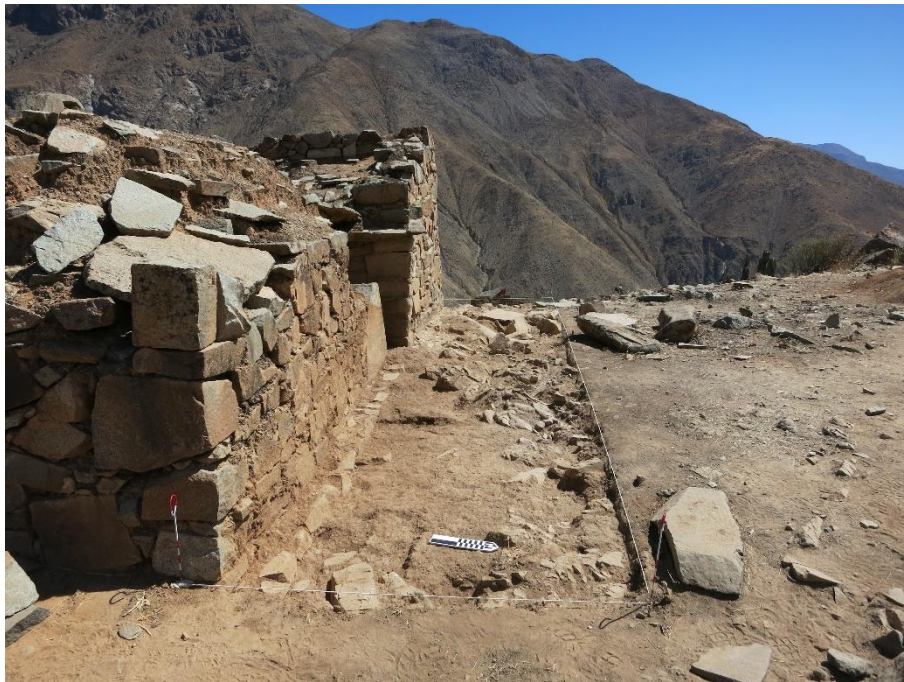
Figure 6.29: Excavation of the trench at the front of the Funerary Area; notice the arrangement of flat stones at the base of Room 1 and bedrock perforating the floor (photograph by PASL 2015).
