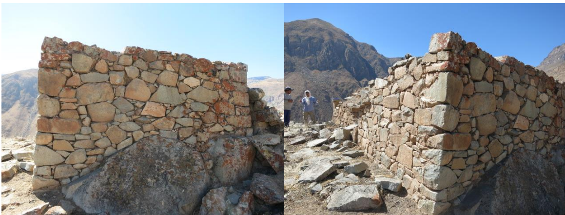
Figure 6.46: Funerary Area. Details of the walls showing the carefully-built masonry. Notice that there is integration of outcrops into the walls, and that the corners of the building are particularly well-angled. There is a careful arrangement and fit within the medium and small stones, even where the mortar is not well preserved. These structures have been dated to the Late Intermediate Period yet are comparable in quality and layout to the Late Horizon-dated structures (photographs by PASL 2015).
