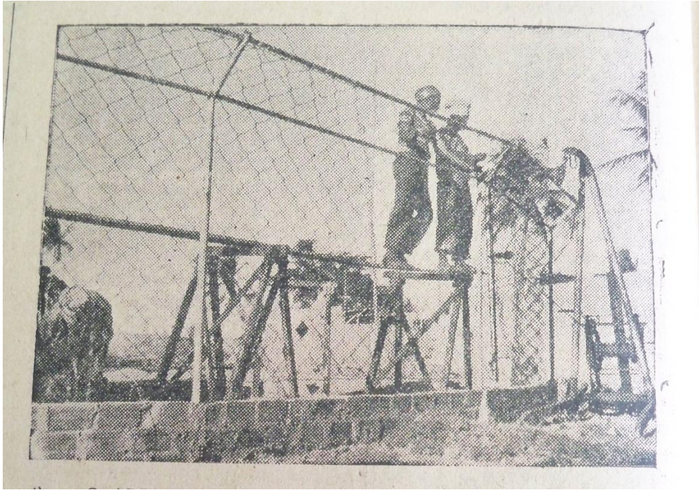
Figure 45: Construction work at the Ilha do Retiro Stadium
