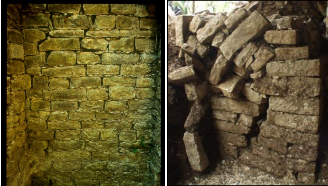
Figure 11.1 Hard limestone masonry walls (Photos by T. Barrientos, VCAP)
