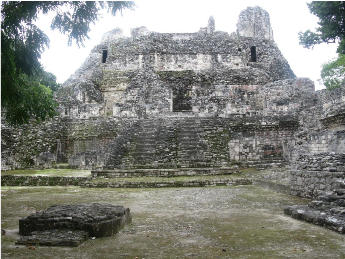
Figure 8.53 North façade of Structure IV, Becán (Photo by T. Barrientos)
