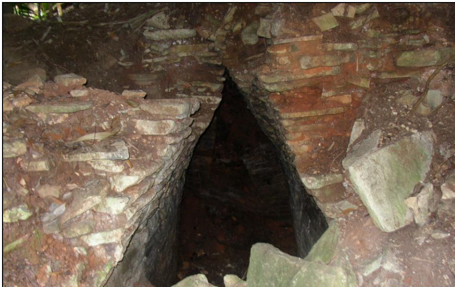
Figure 11.2 Hard limestone vaults made with thin stones (Photo by M. Callaghan, VCAP)
