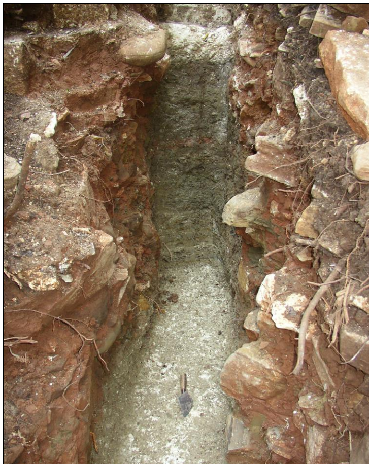
Figure 11.10 Reddish clay used as mortar in stone masonry constructions (Photo by M. Callaghan, VCAP)
