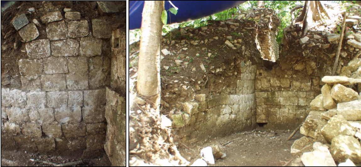
Figure 9.20 Excavation of Southwest corner of South Patio, Northern façade, Structure L7-9 (Photos by T. Barrientos, VCAP)
