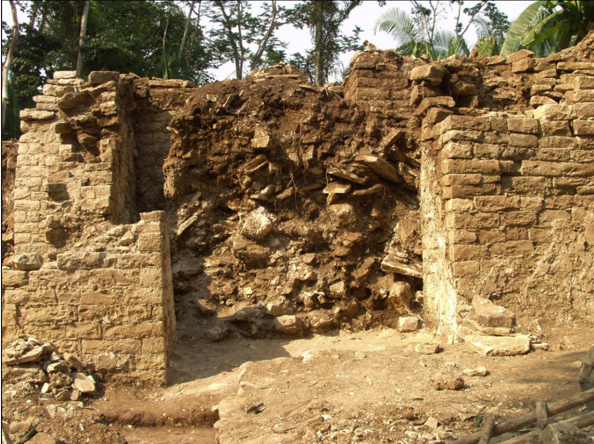
Figure 9.38 Restored entrance of Room 3, northern façade, Structure L7-9 (Photo by T. Barrientos, VCAP)
