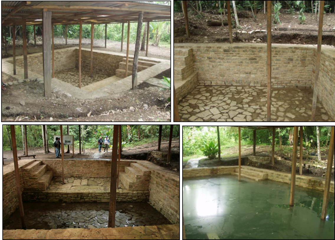
Figure 9.257 Palace Pool restored (Photos by T. Barrientos and L. Luin, VCAP)
