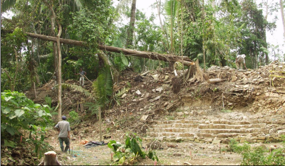
Figure 9.56 Cutting the tree above the Central Corridor of Structure L7-9, during the 2003 field season (Photo by T. Barrientos, VCAP)
