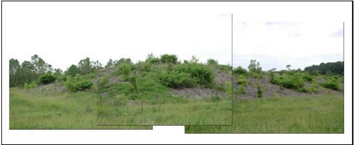
Figure 37. Photograph of Burrell UMTRCA Disposal Cell illustrating vegetative community present on riprap cover.
