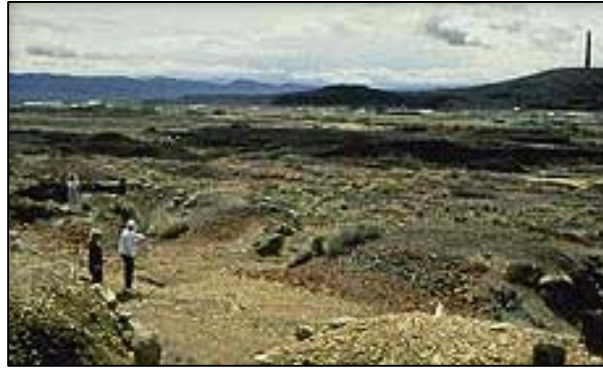
Figure 8. Construction of the Old Works Golf Course (Troon, 2004).
