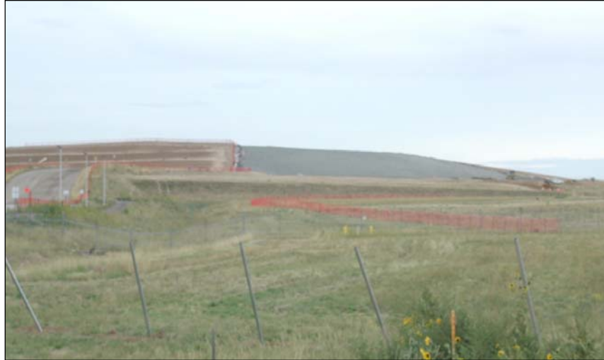
Figure 26. Photograph of RCRA landfill under construction at RMA.
