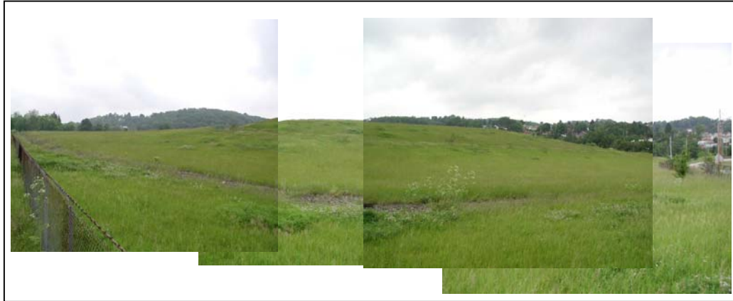
Figure 34. Photograph of Canonsburg UMTRCA Disposal Cell.
