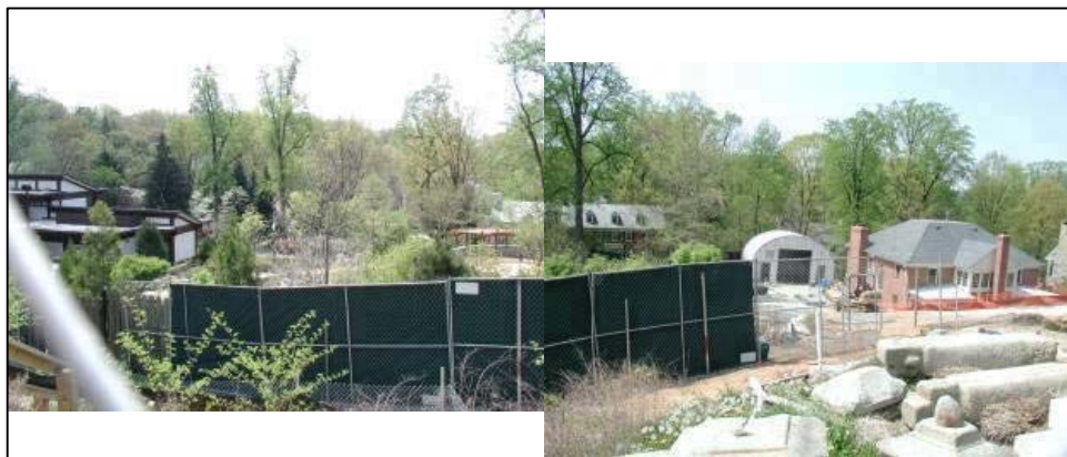
Figure 30. Photograph of remedial operations at Spring Valley.
