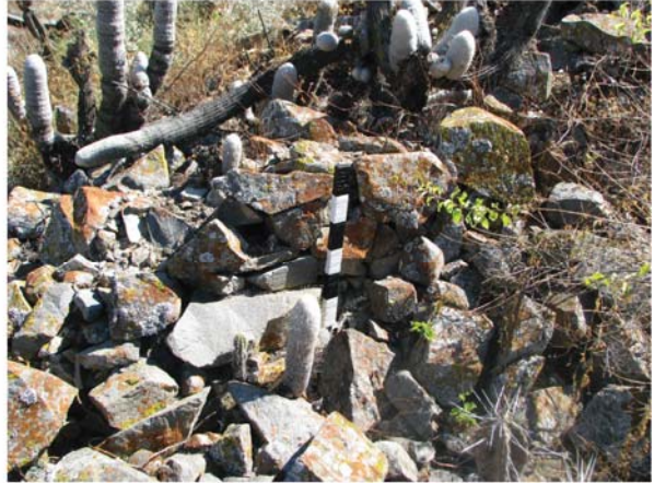
Collapsed structure at Huanangui
