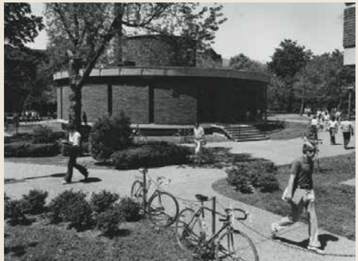
The university housed its computers in the round building that now is the Biomolecular NMR facility.
