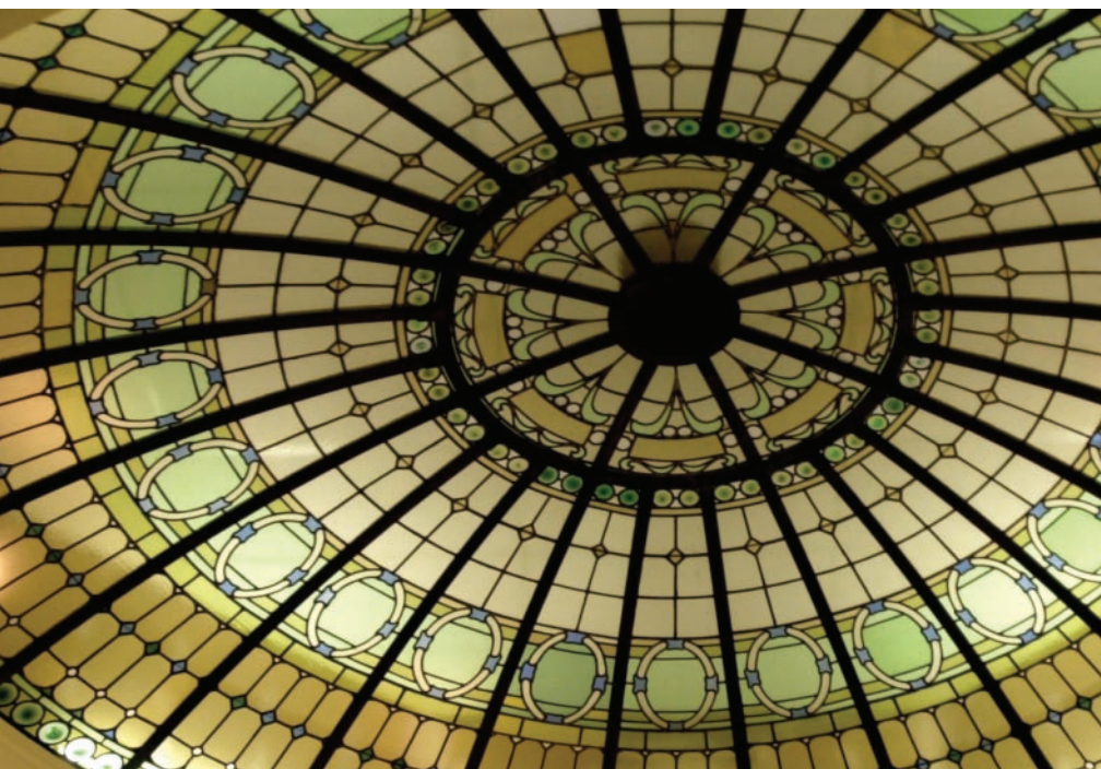
Mayborn Building Skylight
