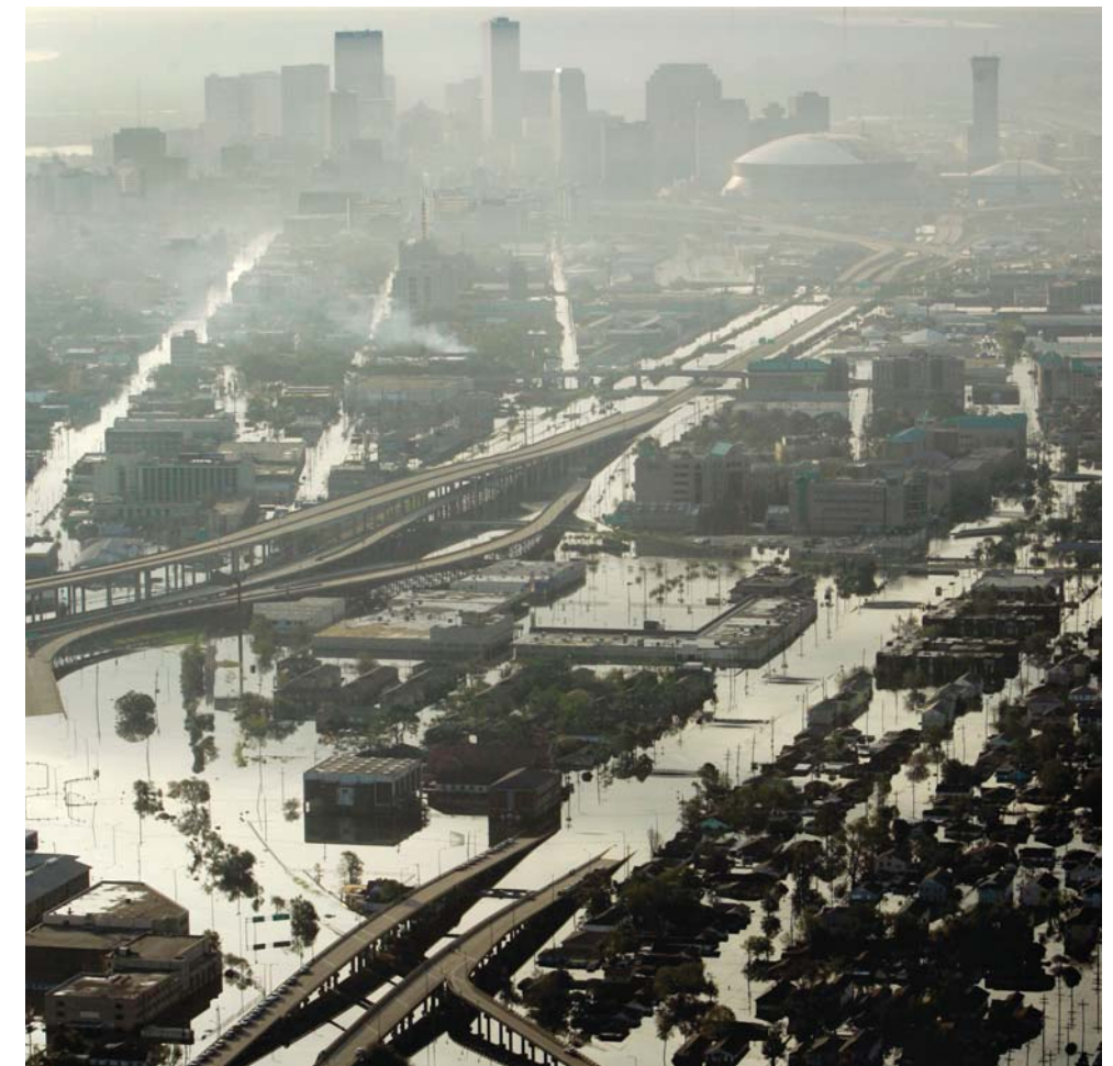
Floodwaters fill the streets of New Orleans, August 30, following Hurricane Katrina.
