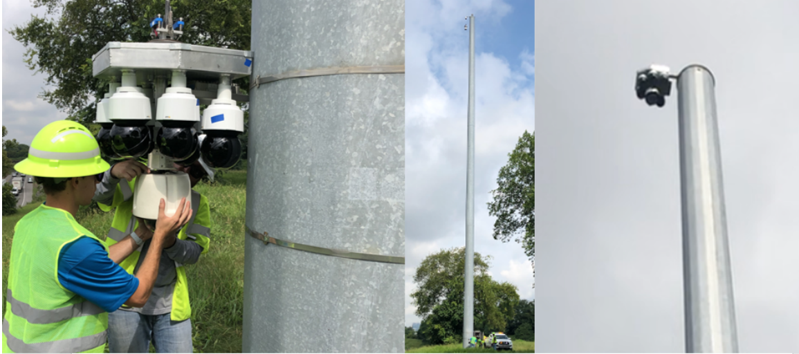
Figure 3.6: Multi-camera mount is raised onto 110 ft pole.
