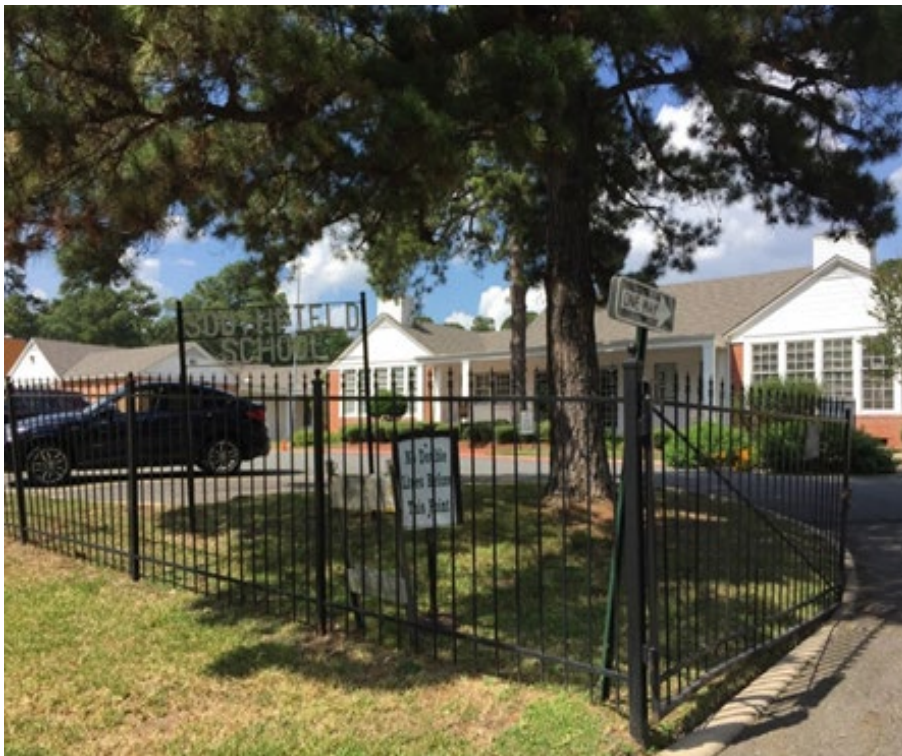
Figure 9: Southfield School facade
