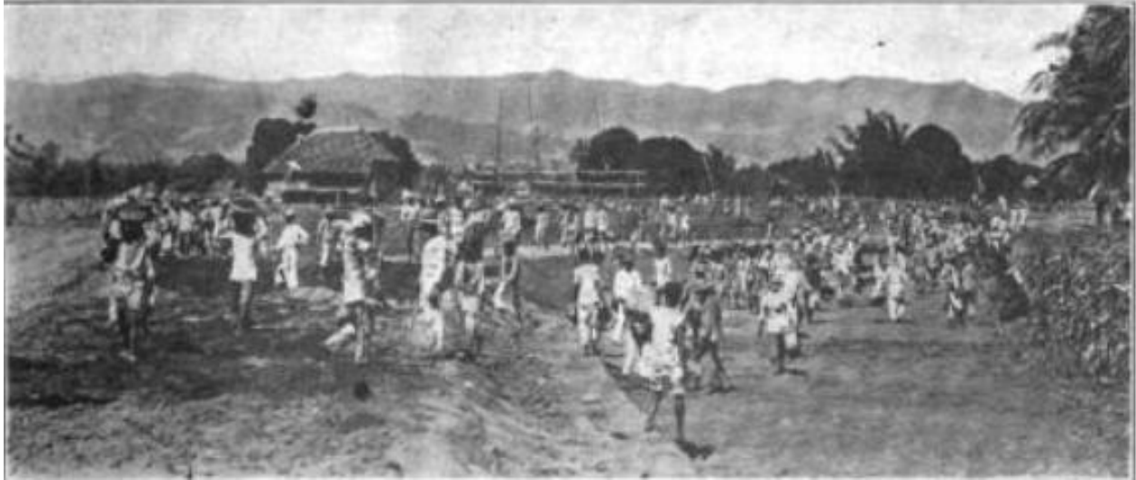
Figure 2-8: Workers Grading Land for Construction of Philippine Railway ( The Railroad Gazette , 1907)
