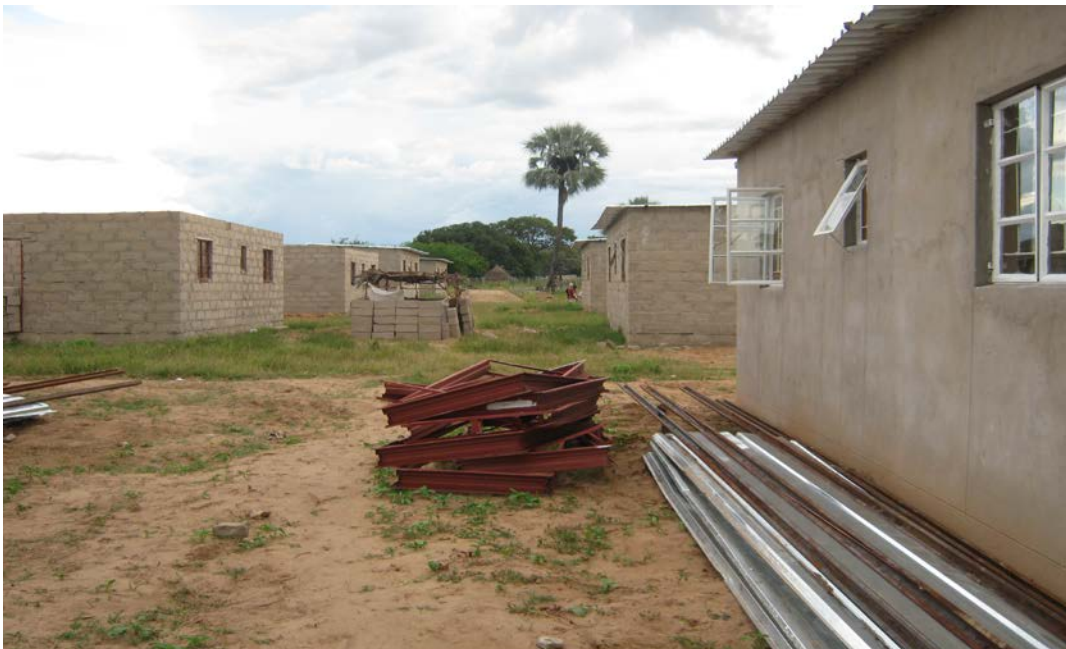
Photo #4: Federation Neighborhood under Construction, Nkurenkuru, Namibia (north-central Namibia), Monday, March 10, 2010.
