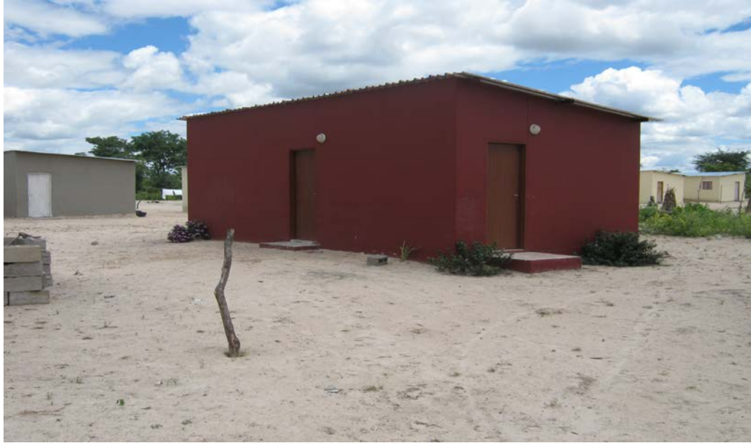
Photo #5: Finished Federation House and Federation Neighborhood, Eenhana, Namibia – Northwest Namibia, near the Angolan border – Friday, March 5, 2010.
