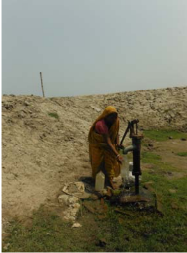
Figure 14. Photo (5/15/12). A Polder 32 inhabitant accesses the shallow groundwater resource through a hand-pumped tube well.
