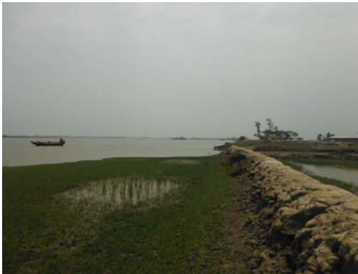
Figure 10. Photo (5/14/12). Shrimp pond developed inside earthen berm (right side of photo) and adjacent to Dhaki River in background.
