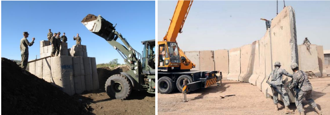
Figure 1.1 Soil-filled barrier construction (left) and precast concrete barrier construction (right)
