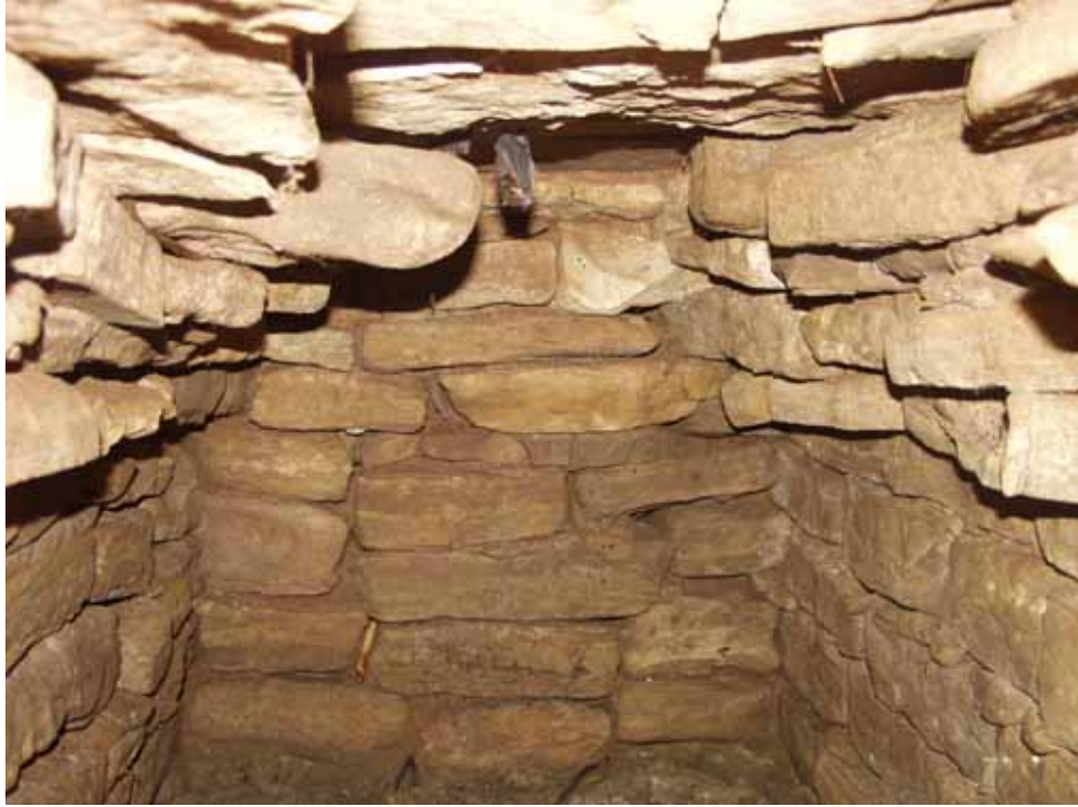
Figure 9.7. Vaulted tomb in Structure N10-1 (photo by author).
