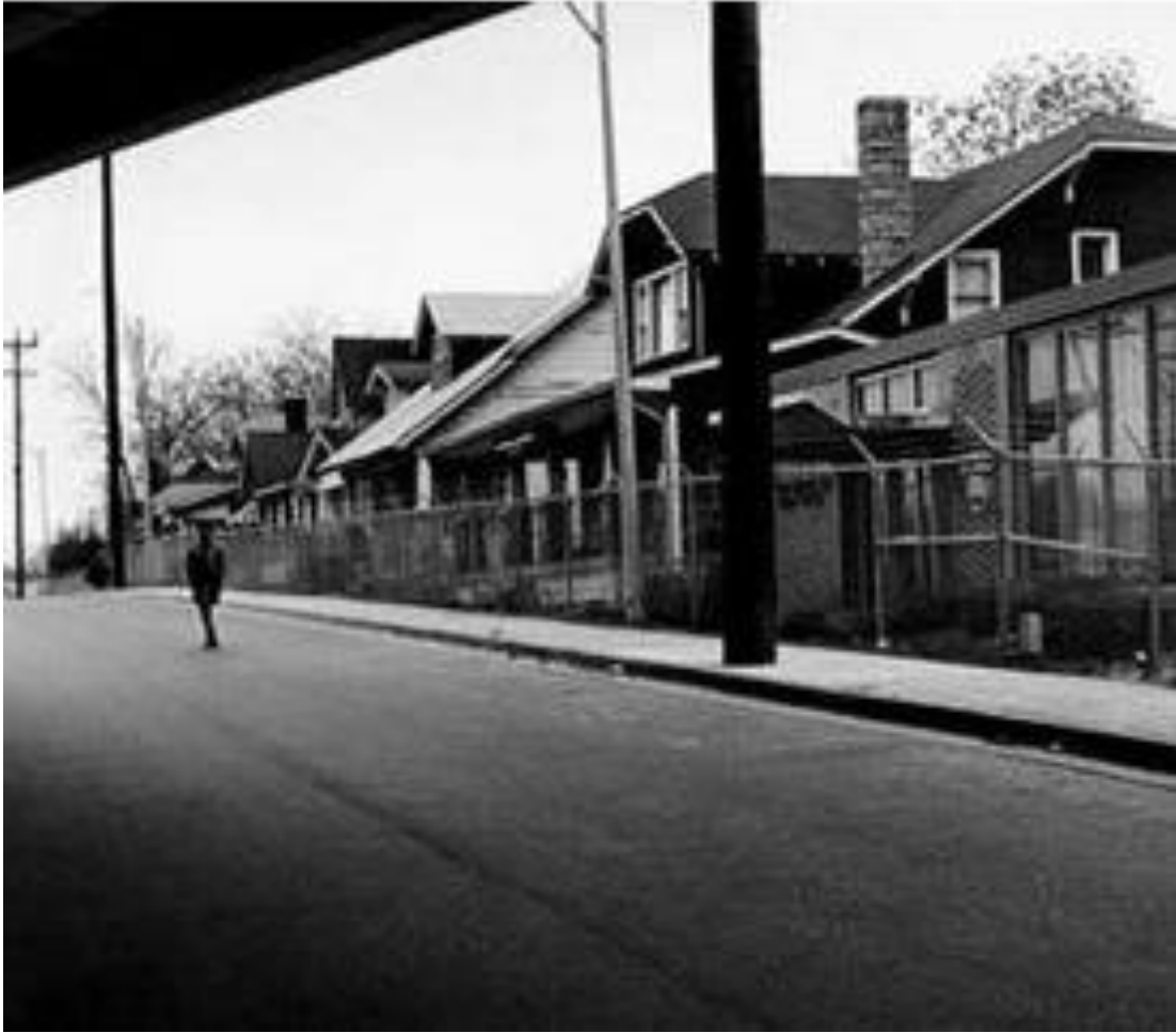
Figure 7: This image from 1970 shows 6 foot tall fences that were erected around the homes and businesses during the time of construction. Ellis, Jimmy. 1970. The Tennessean, Nashville. Tennessee 4 Me-An African American Community's Fight over I-40. Web. 9 Dec. 2015.
