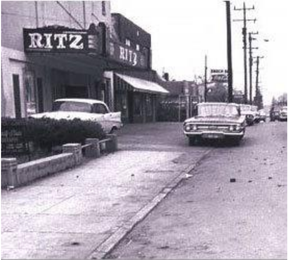
Figure 6 A photograph of the Ritz Movie theatre before it closed down because of highway construction. N.d. Metro Nashville Archives, Nashville. Tennessee 4 Me-An African American Community's Fight over I-40. Web. 9 Dec. 2015.
