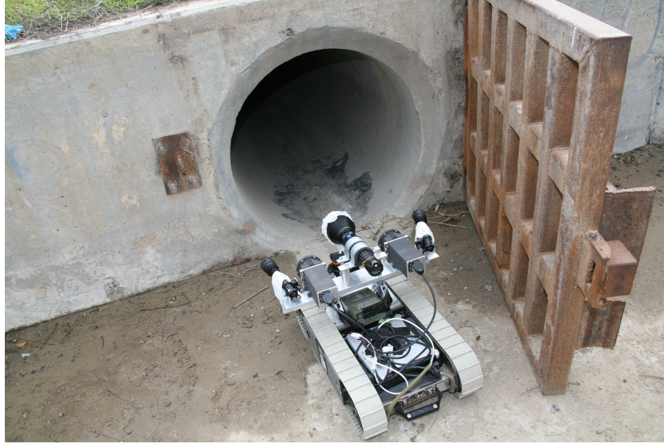
Figure IV.3: Border tunnel robot
