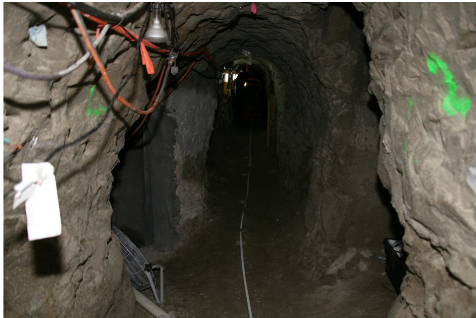
Figure IV.2: Tunnel Experiment Smuggling Tunnel
