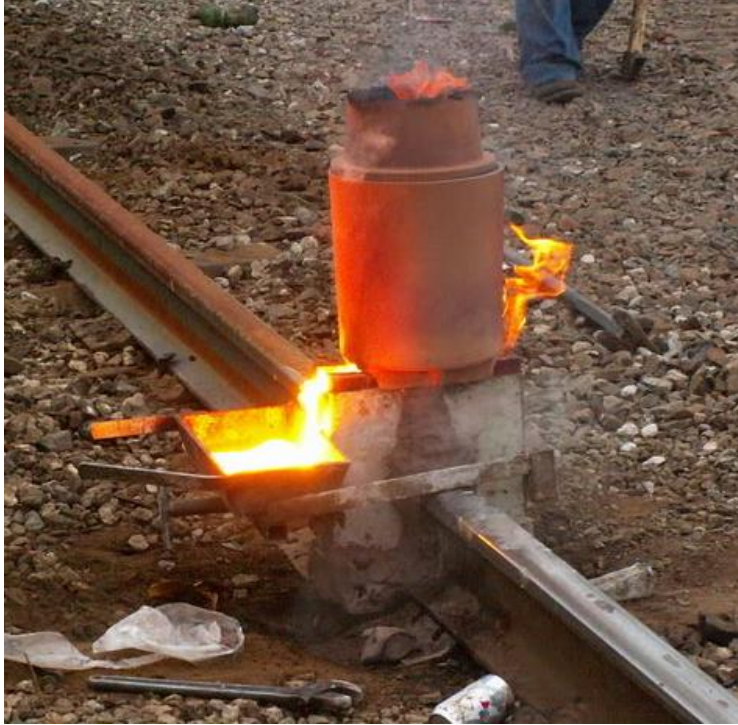
Figure 2 – Thermite Welding on Railroad Tie [5]
