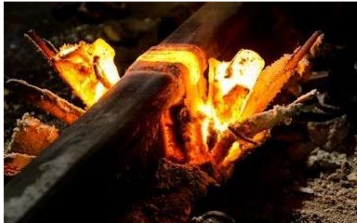
Figure 3 – Completed Thermite Weld [3]
