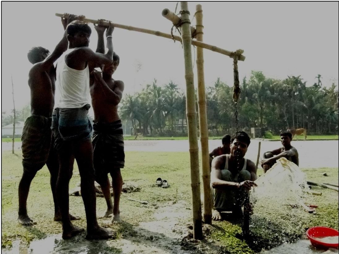
**Figure 7. This hand driven reverse circulation drilling technique is an economical and efficient method for sample collection from the unconsolidated fluvio-deltaic stratigraphy in Bangladesh.**
